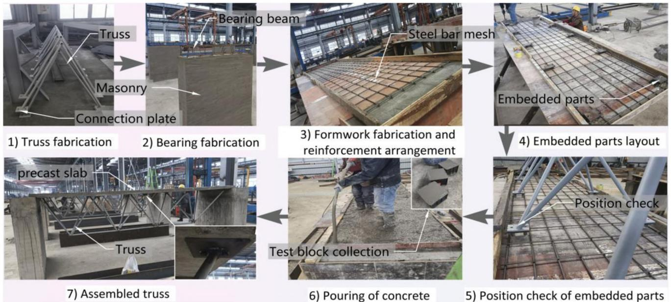
Figure 5 Construction process of the experimental model.
