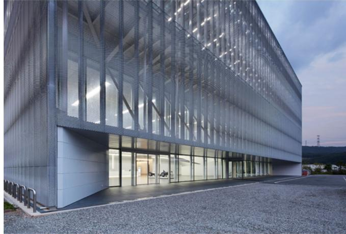
**Figure 2:** Expanded Metal Façade Cladding at Hyundai Motor Training Center, South Korea.
