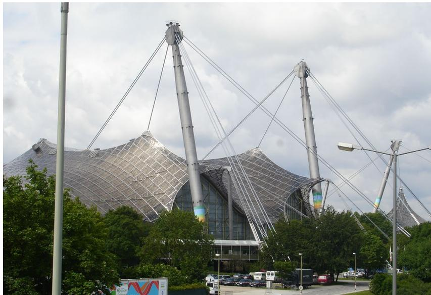
**Figure 1:** Tensile membrane structure in the Olympia Park at Munich, Germany. (image by J. F. Valdés-Vázquez)
