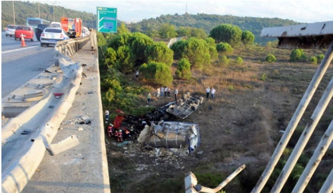
*Figure 2. Bridge rail failure due to a heavy vehicle impact in Istanbul [Atahan, 2016]*
